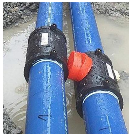
Figure 2-16: The pipes are connected by electrofusion
