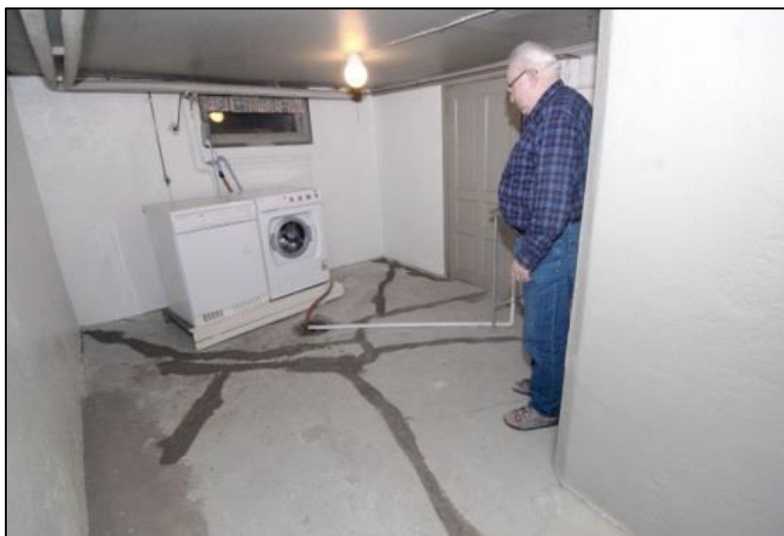
Figure 4-6: Damages in basement in Solna, Sweden
