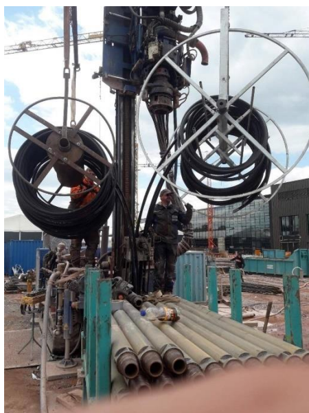
Figure 2-9: Reels are being unrolled during the pipe installation
