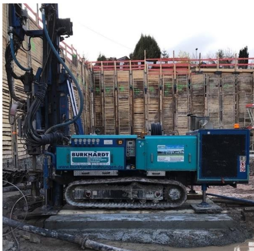
Figure 2-2: The drilling rig is placed on a platform, which was installed specially for this purpose
