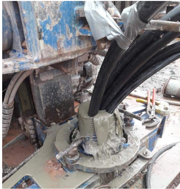
Figure 2-12: During the installation process the drill hole is flooded
